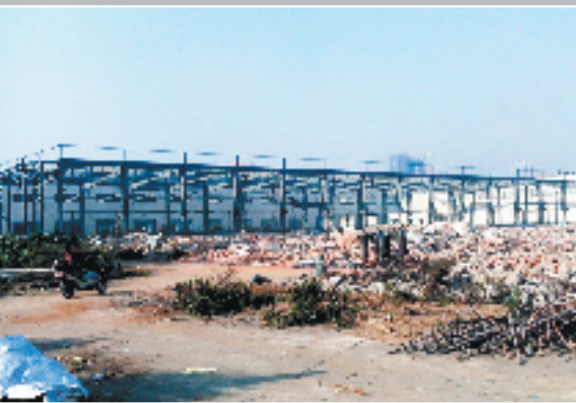
诸暨市陶朱街道违建厂房拆除前
